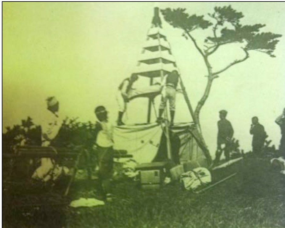
Figure 2. Surveyors constructing a signal pole atop a Korean peak. Source: GGK (1911 40).
